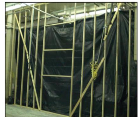
Temporary barriers can protect the production environment from aerosols and traffic that may carry Listeria exposed during construction.
