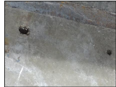
Holes from equipment that has been moved should be sealed to avoid harborage areas
