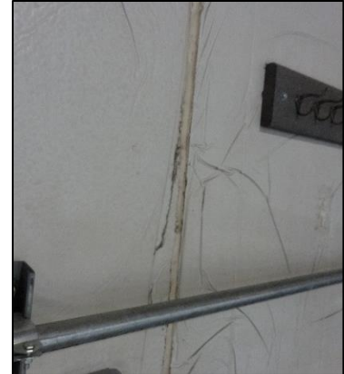
Cracked and caulked walls are common harborage points for Listeria
