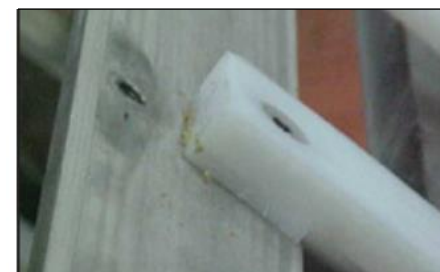
Avoid overlapping materials where joints cannot be sealed
